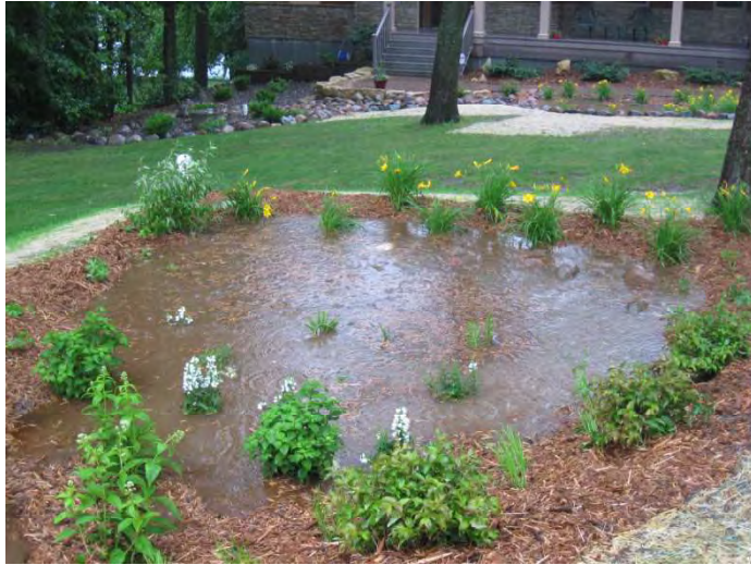
Figure 62. Rain Gardens Collect and Infiltrate Runoff Water in this Deer Lake Rain Garden (photo by Steve Palmer)
